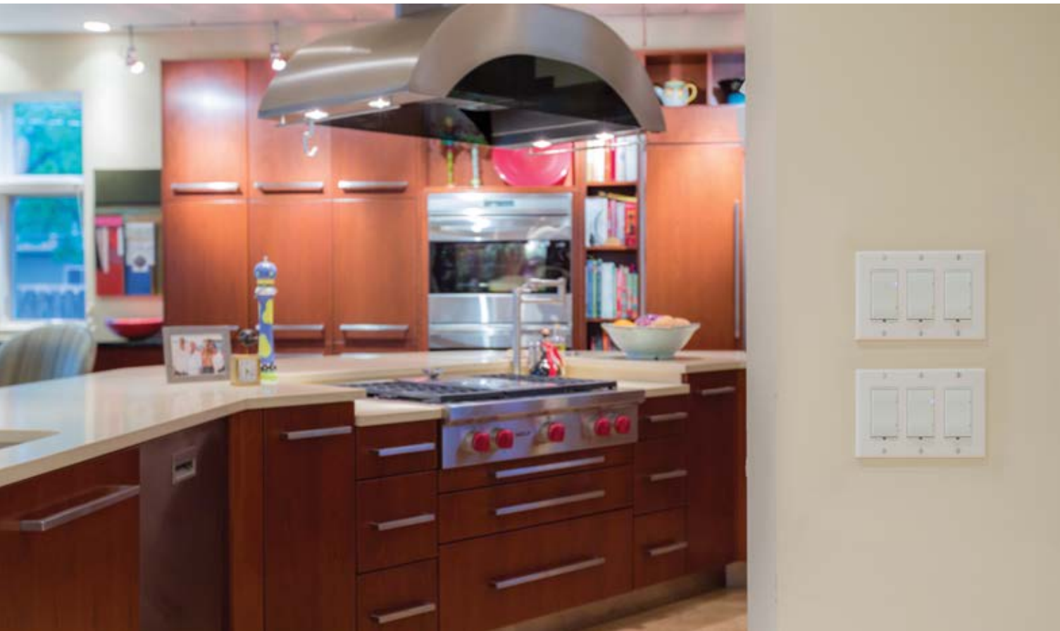
Program a button to turn on all the lights in the kitchen to full brightness, and label it COOK.
