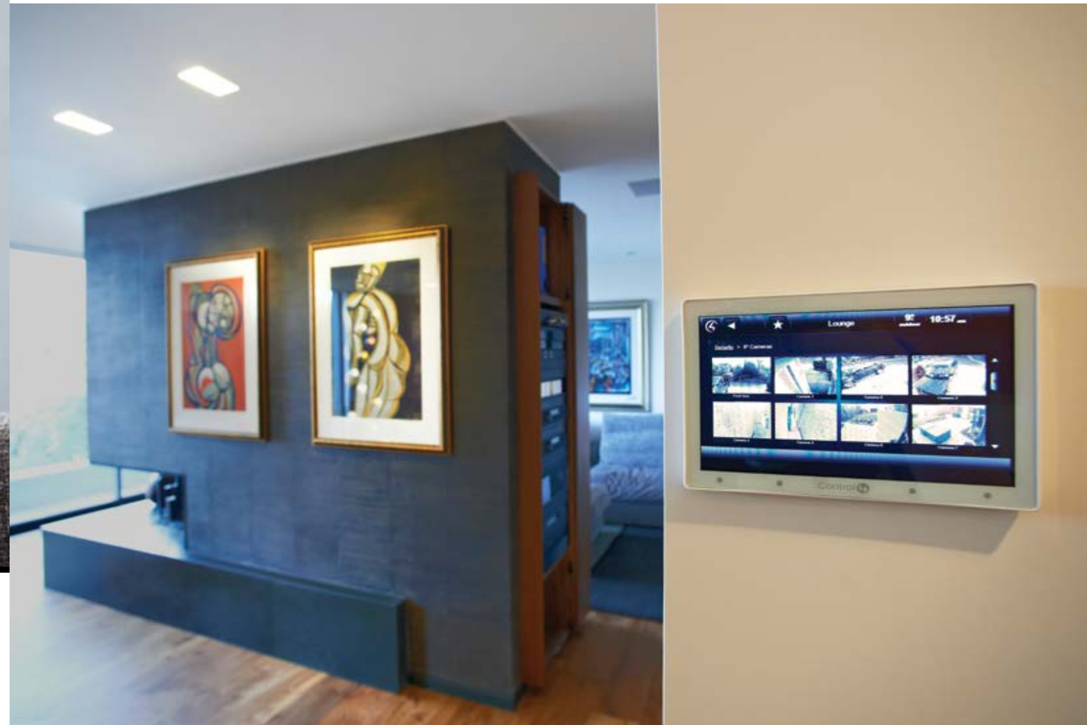
A perfectly positioned touch screen makes it easy to monitor the whole home from one location, and control the fireplace, adjust the lights, and so on.
