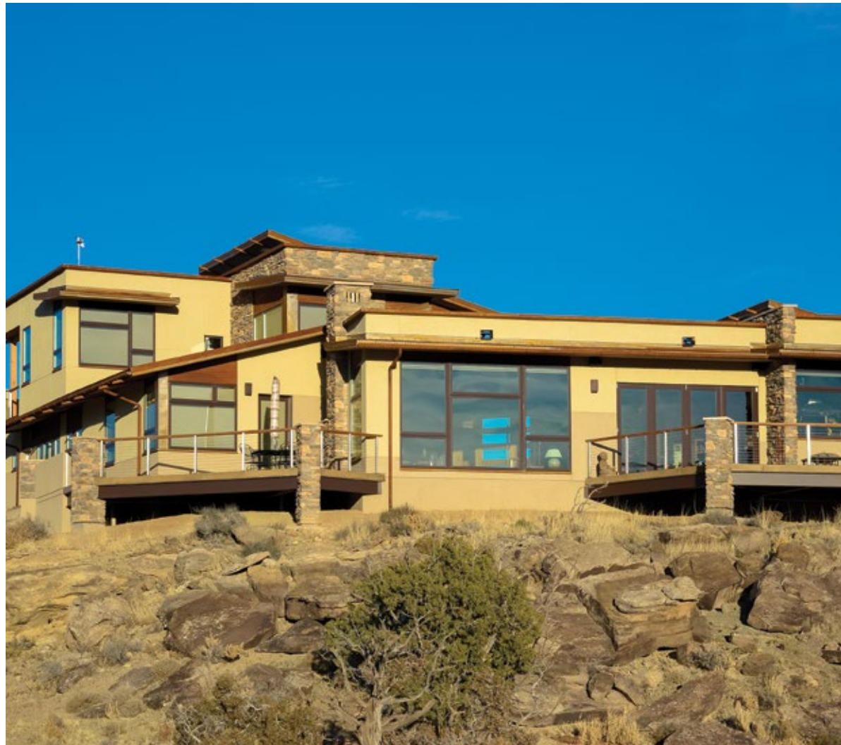
The 3,000-square-foot “high desert modern” house appears as if it grew out of the hillside. Lots of windows provide sweeping views and help regulate indoor climate with motorized shades.
